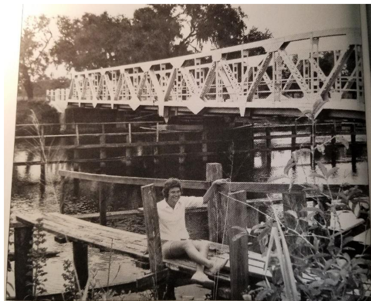
Until a barge full of rocket parts bound for the Kennedy Space Center crashed into it in 1966, the Alva swing bridge lent old Florida charm to the town's landscape. (HFA.)
