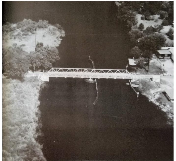
Until 1966, Alva had a swing bridge instead of a drawbridge. When a boat needed to pass, a section of the bridge would rotate open to allow the boat passage through the bumpers on the right side. (US Army Corps of Engineers.)
