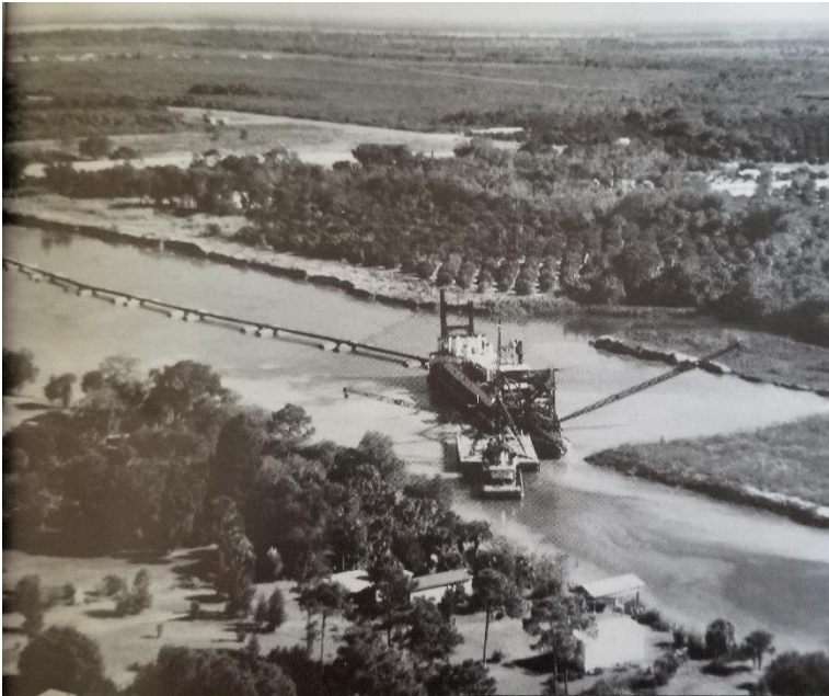
The Caloosahatchee has undergone many bouts of dredging and straightening since the 1800s. In the 1960s, the river was widened and deepened. This photograph, taken near LaBelle, shows the massive dredge with the boat behind it from which spoil material was pumped into floating pipes and deposited as much as half a mile from the river. (Author's collection.)
